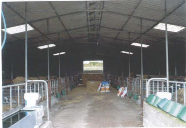
Figure 2. Inside the calf housing shed.
