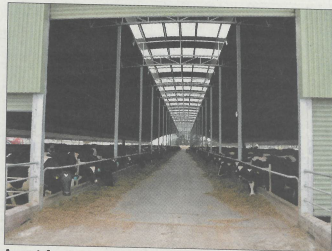
A new infrastructure being built to house cows for longer periods.
